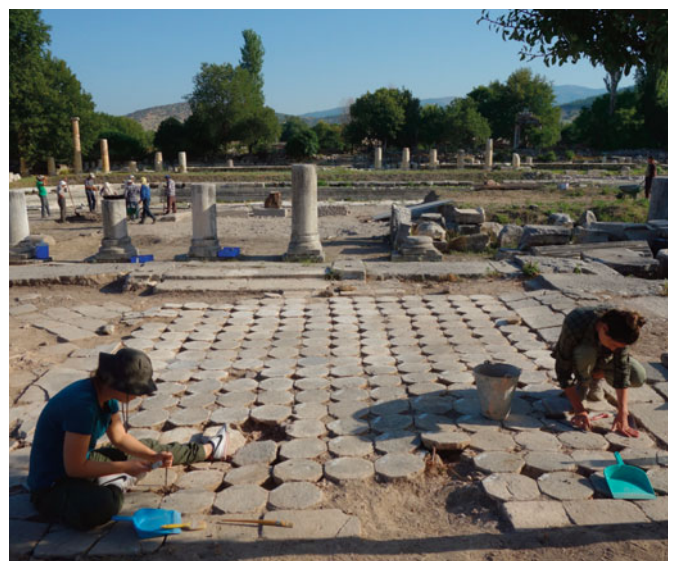
Conservation of the marble-tile floor in the Basilica.
