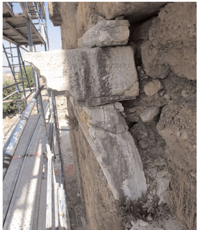
A decorated architrave frieze block, revealing the limestone block on top of the cornice as well as the row of limestone blocks below the architrave (forefront of photo). The mortared rubble connecting the decorated building elements and the conglomerate back wall is also clearly visible
