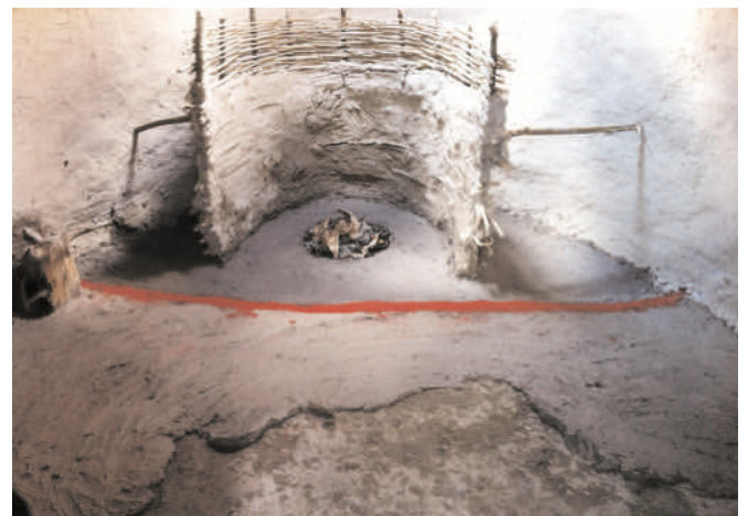
Replastering and painting the floor of an experimental house
