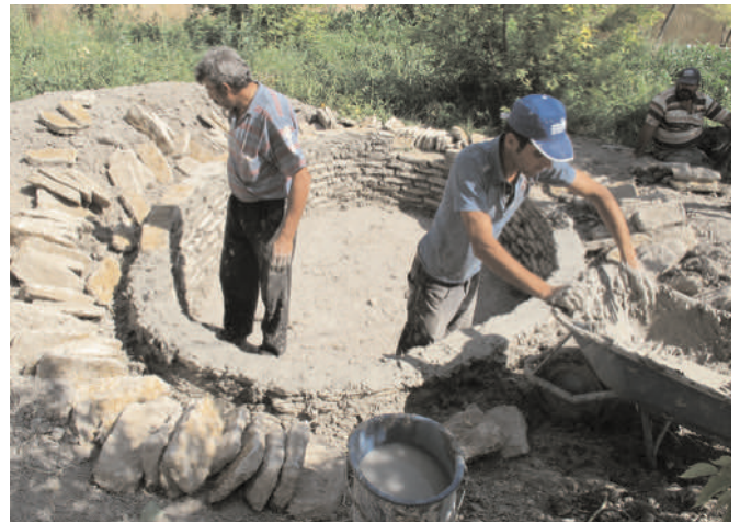
Boncuklu experimental house 1 under construction.
