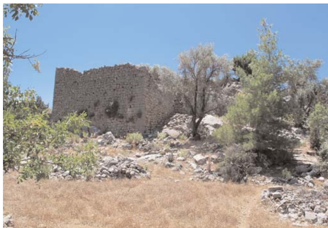
View of the remains at Yumaklar, Bekirler Kalesi
